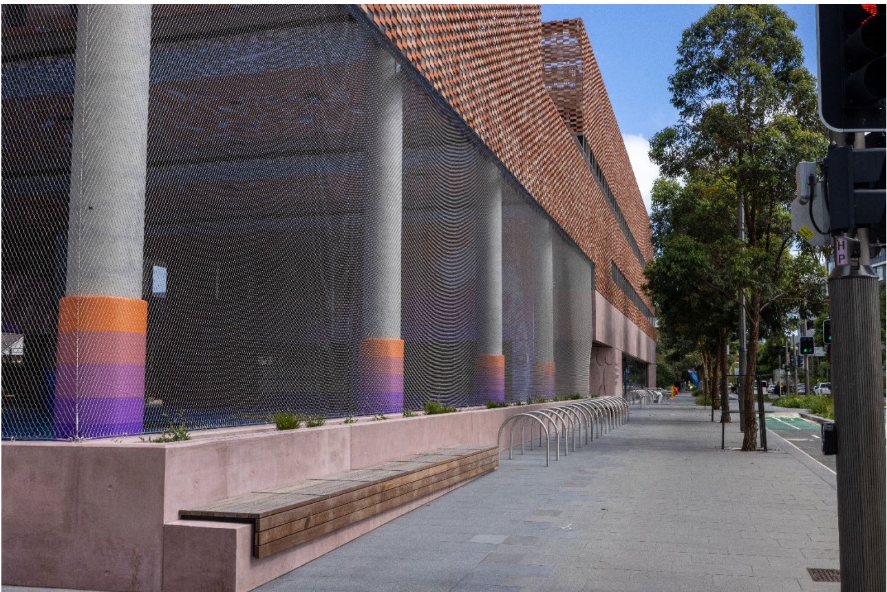
Figure 7. Green Square public school and community spaces, Green Square – jointly funded by NSW Government and City of Sydney. Abril Felman/City of Sydney
